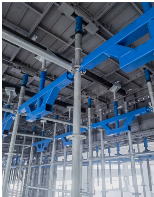
Reinforcement Scheme for Slab Panel with Heavy Loads 大荷载顶板加强方案
