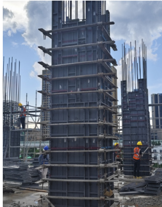
Column Formwork Solution 2 柱模解决方案二
